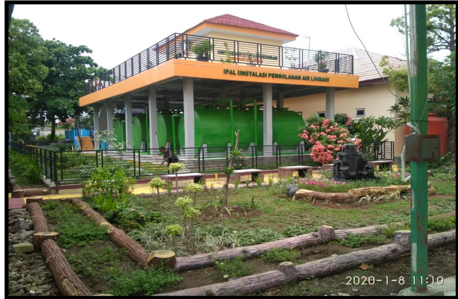
Gambar 3.42 IPAL RSUD Indramayu
